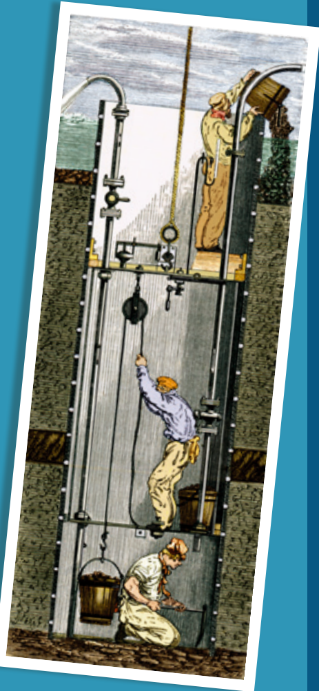
Les 3 compartiments du procédé Triger - The 3 compartments of the Triger process
